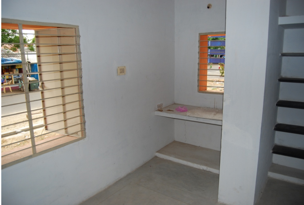
Separate Toilet constructed in the house
